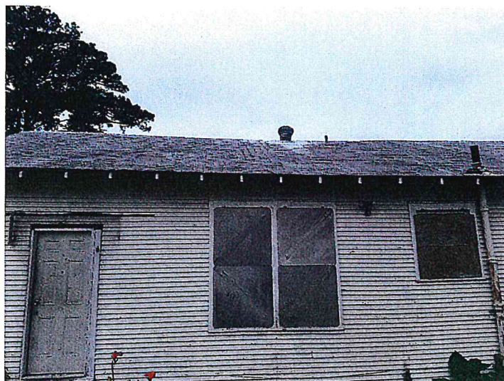
4/19/2016 SAMPLES S59 & S60 - SHINGLE ROOF & FELT MTRL Pic (16).jpg
