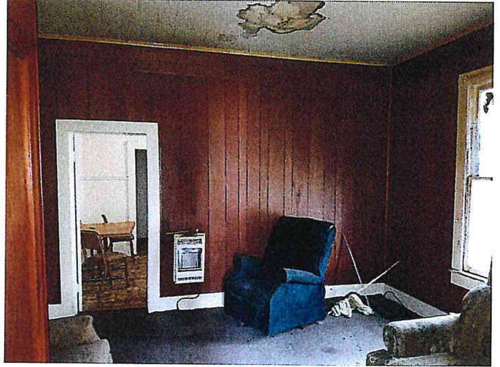
4/19/2016 416 A&B - INTERIOR B SIDE Pic (10).jpg
