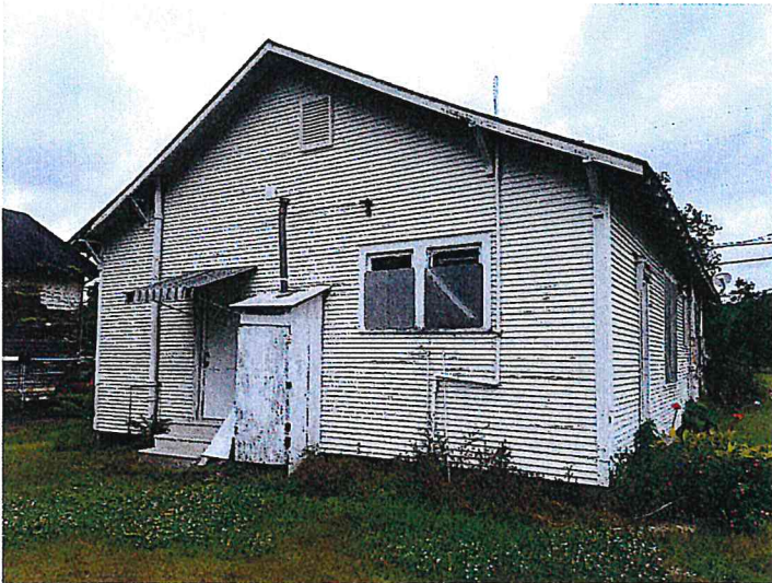
4/19/2016 EXTERIOR SIDE C - 416 A&B MUDD STREET Pic (03).jpg
