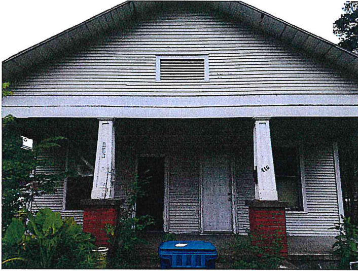
4/19/2016 EXTERIOR SIDE A - 416 A&B MUDD STREET Pic (01).jpg
